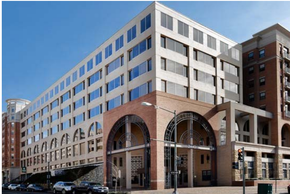
Harrison Street paid more than $500 million for medical-office buildings in the Washington area. James Oesch
