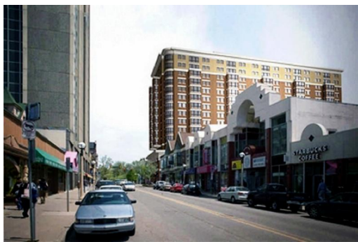
A rendering of Harrison Street's $75 million, 650-bed development in Ann Arbor, Mich., adjacent to the University of Michigan campus. Photo by: Harrison Street
